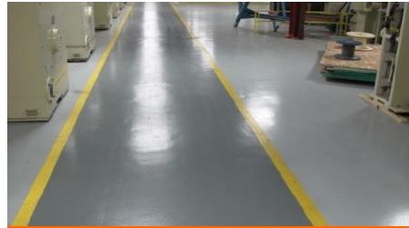
CONCRETE DUST PROOFER APPLICATION
