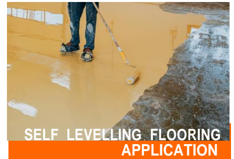
3D.EPOXY.FLOORING INSTALLATION
