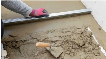
STANDARD FLOOR SCREEDING APPLICATION
